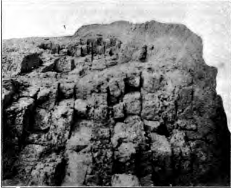
CRUMBLING WALLS OF REI
